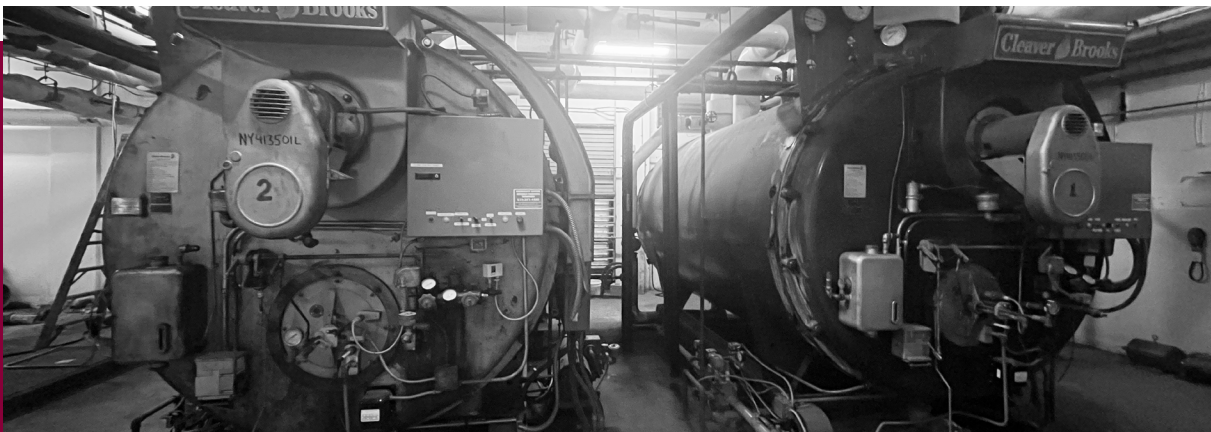
Old Boiler Old boilers are either “all on” or “all off,” which leads to inefficiencies when the weather is merely chilly rather than downright frigid. Approval of Proposition #1 would upgrade components of the High School’s boiler system to improve energy/cost efficiency and reliability.
